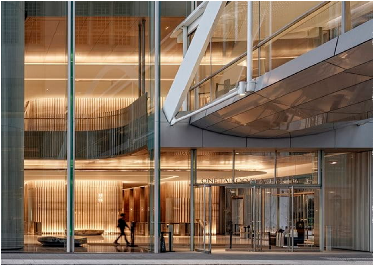
Street Level Entrance to the Building with step free access
